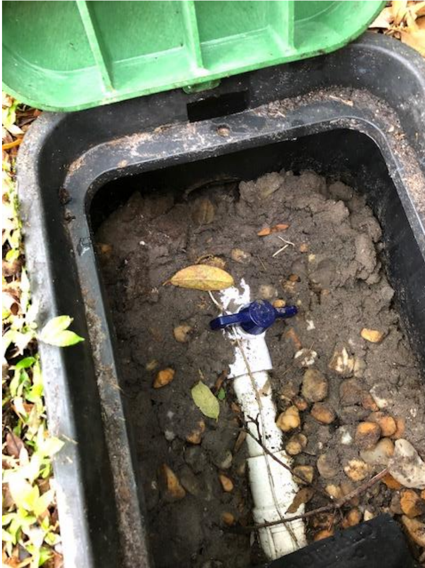
Image 3 – West Side Irrigation Valve shutoff in the OFF position
